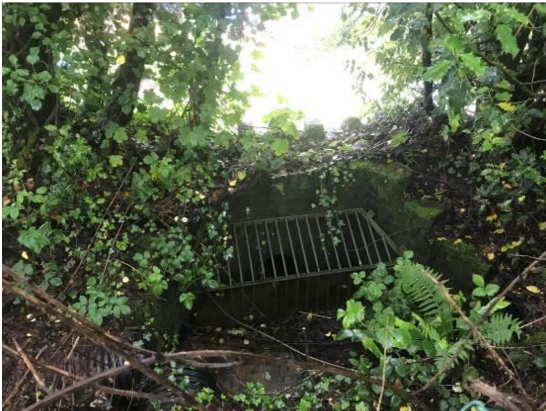
Photograph 36 – Inlet chamber at rear of school
